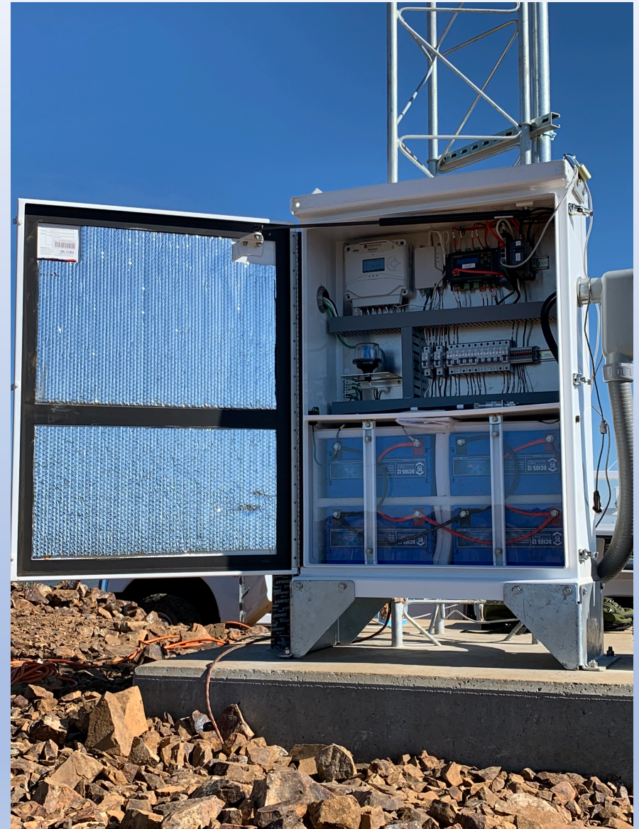
Enclosure with 400 Ah of batteries
