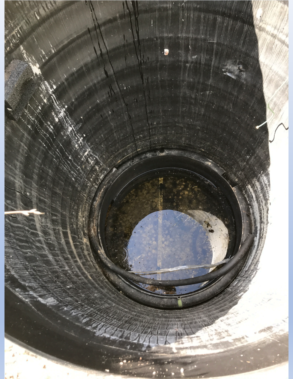
Flooded TA vault with 6" of water
