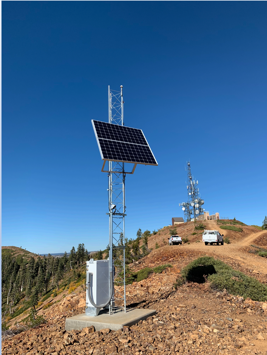
Solar panels elevated for snow loading
